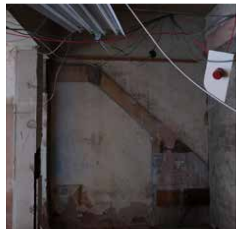
Evidence of past staircase (Ground Floor)
