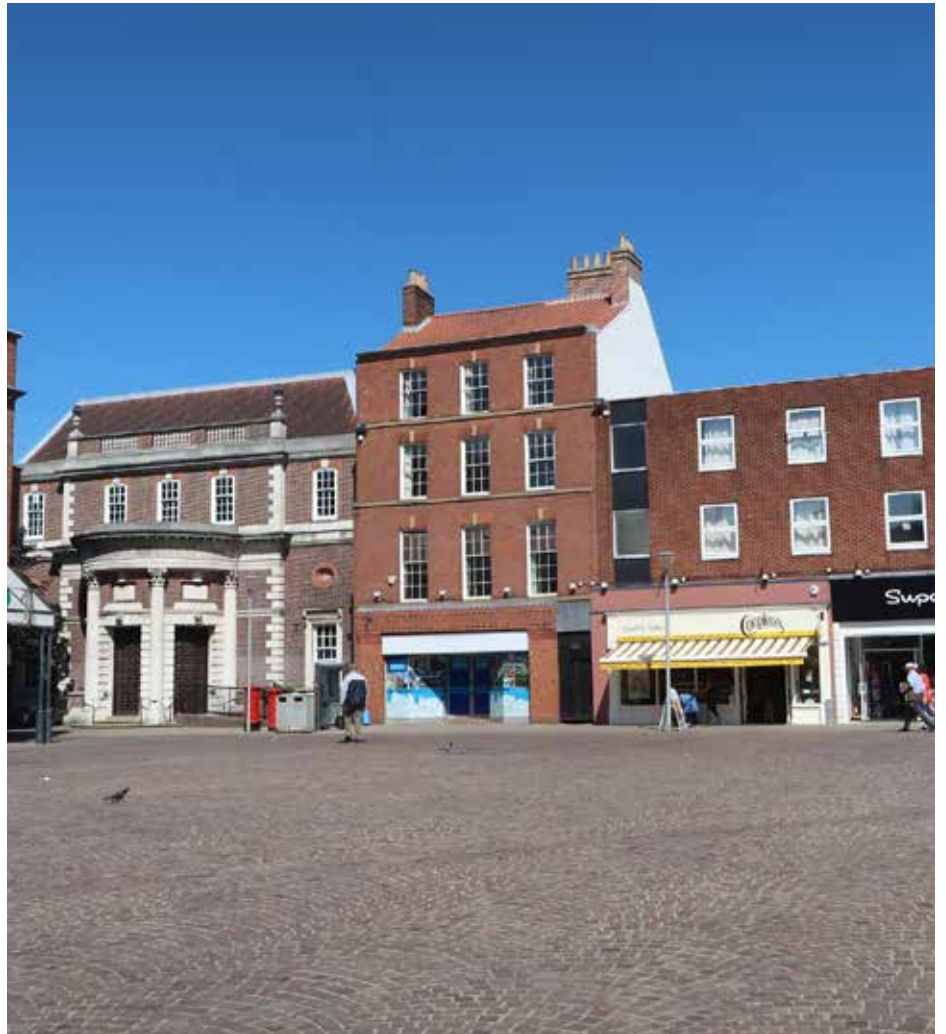
5-7 Market Place with the former NatWest Bank to the left (North)
