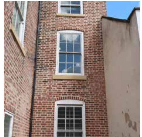
Evidence of replaced lintels
