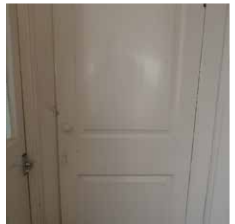
(ix) Cupboard on landing
