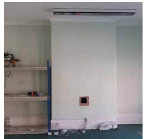
(v) Chimney breast
